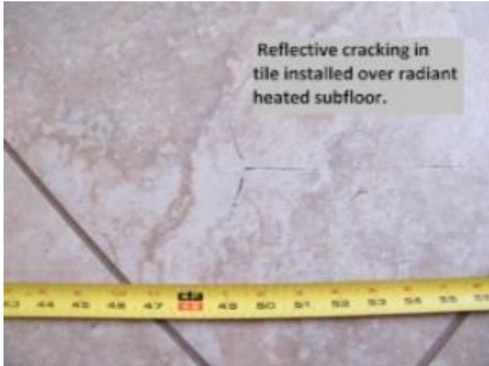
This photo shows a cracked ceramic tile. The crack occurred directly over the OSB subfloor joints. Radiant heat tubes are installed directly to the underside of subfloor. The radiant heat system rapidly overdried the subfloor causing the sanded flat joints to shrink and pull anything installed over it down with it, and when the floor shrunk in thickness it caused reflective cracking in the tile.
