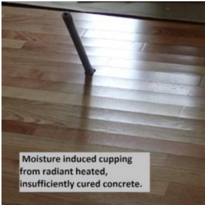
This one is a head shaker and I think someone needs dope slapped. What was the installer thinking? The concrete was less than 60 days old when the installer decided to install this floor over radiant heated concrete. The radiant heat drove the moisture out of the concrete up into the wood. The wood is ruined, very sad.
