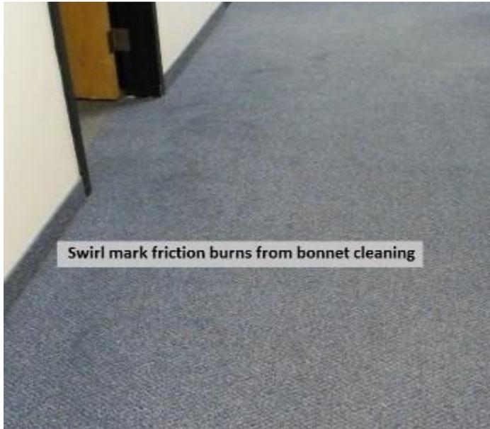
In my last article about bonnet cleaning I used this photo. I have seen swirl marks and crescent-shaped friction burns in carpet because the operator was not using sufficient detergent to lubricate the bonnet. Too much friction between the bonnet and the carpet melted the carpet yarns.
