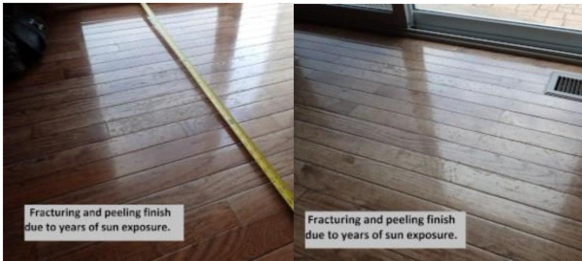
I am certain this floor was lovely when it was first installed 10 years ago. After years of direct sun exposure through the patio doors the finish on the floor is finally giving up and can't take it anymore. Remember polyurethane finishes on wood floors are plastic with ultraviolet light inhibitors but they can only take so much abuse. They eventually become brittle, fracture and disintegrate.
